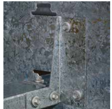
BRIDGE BAR STABILISER Prevents purlin roll
